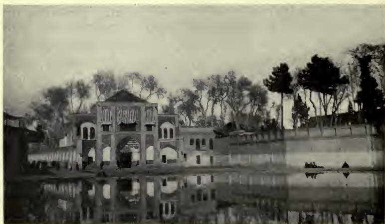
Exterior view of the Palace grounds.
